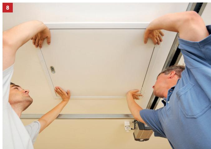
**Placing the loft ladder into the construction opening**
